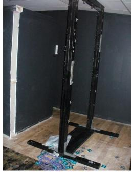
3. A steel cage with three sides, a top and three opening doors on the front, 2000 mm high x 1000 mm deep x 680 mm wide, bolted to a plywood base 1200 mm x 1770 mm, painted black.
